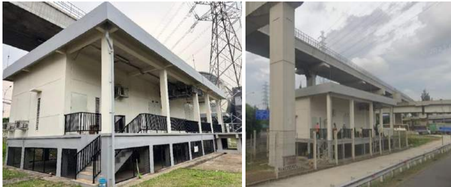
Gambar 7- 30 Traction Power Substation (TPSS)
